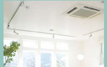
Air Conditioner Units
